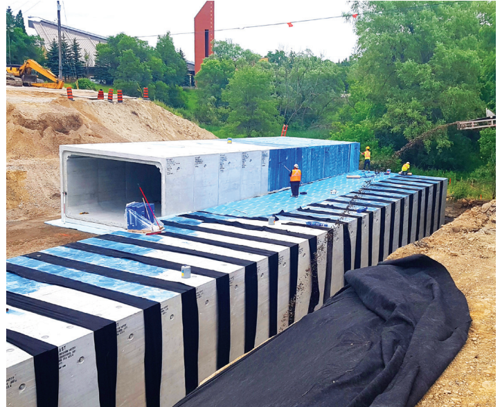
Waterproofing and backfilling
