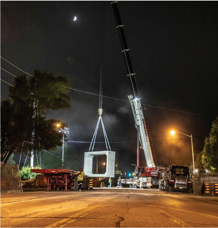
Night culvert installation
